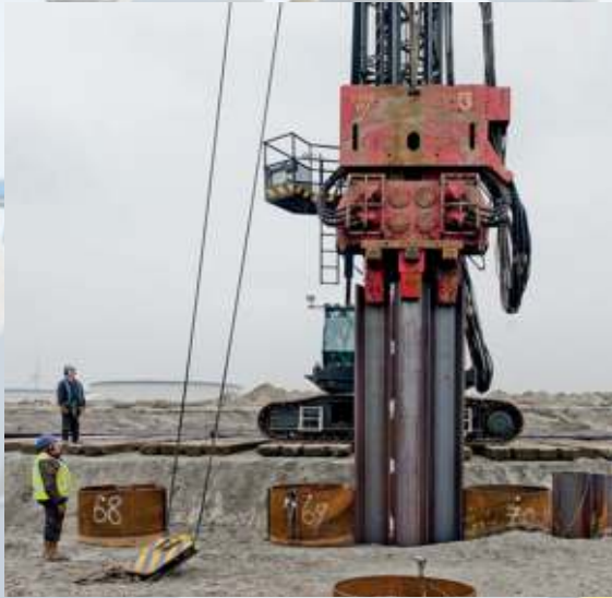
Pile driving machine
